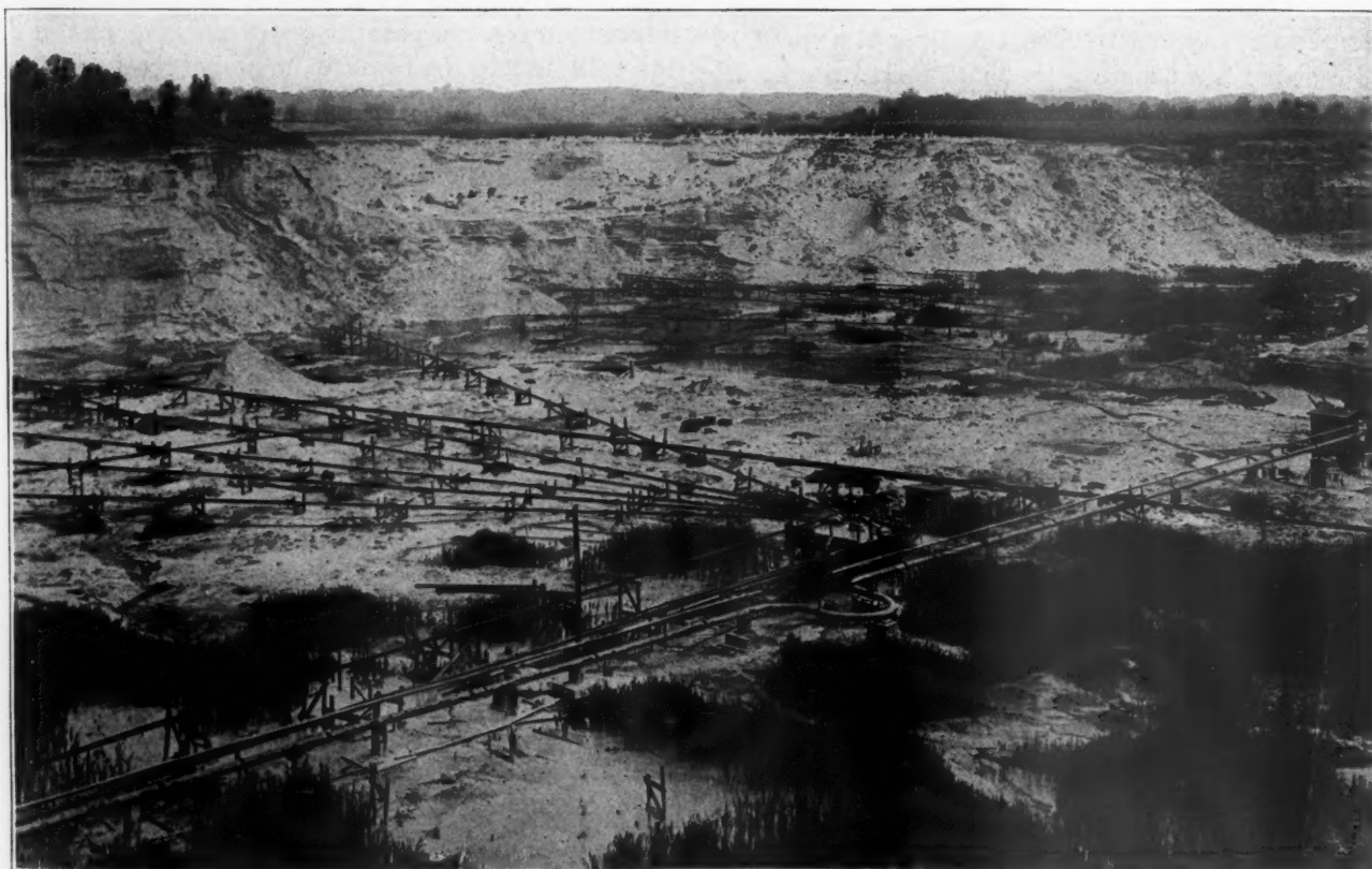
View Showing Layout of Pump Lines From Different Deposit Faces
